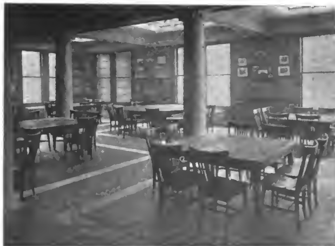
THE GRILL ROOM, WHICH ACCOMMODATES 300 PEOPLE.
